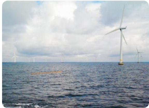
Figure 8: Rødsand II. 90 windmills, 207 MW, 75–80 km cables, area of 34 km 2 plus surrounding restricted area.
